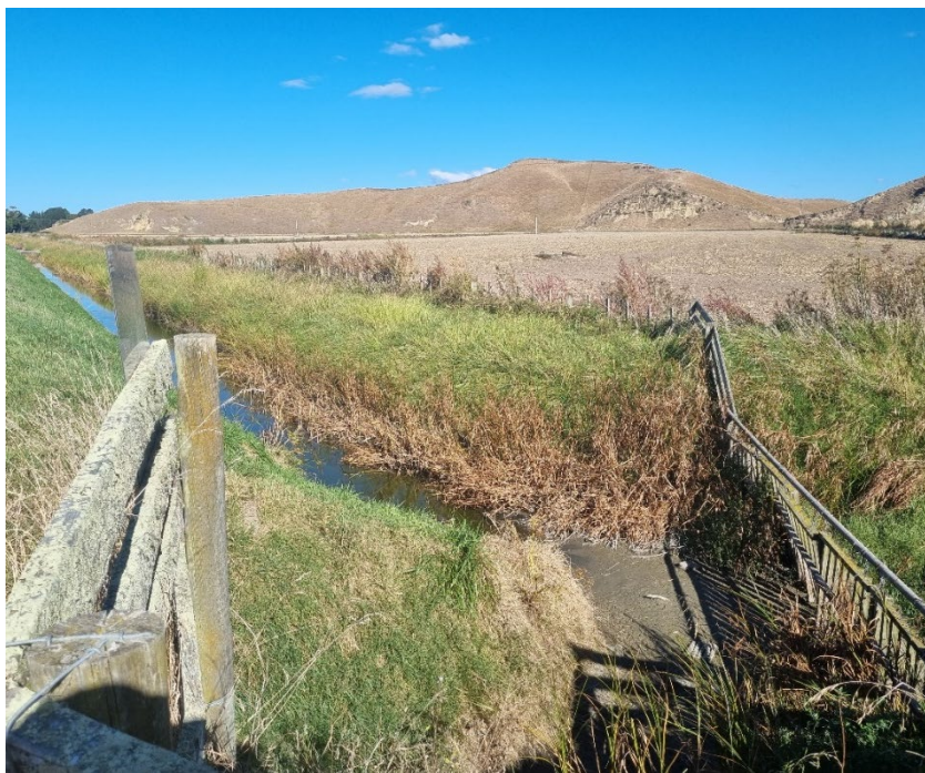
Photograph 17: T5 in dry weather
