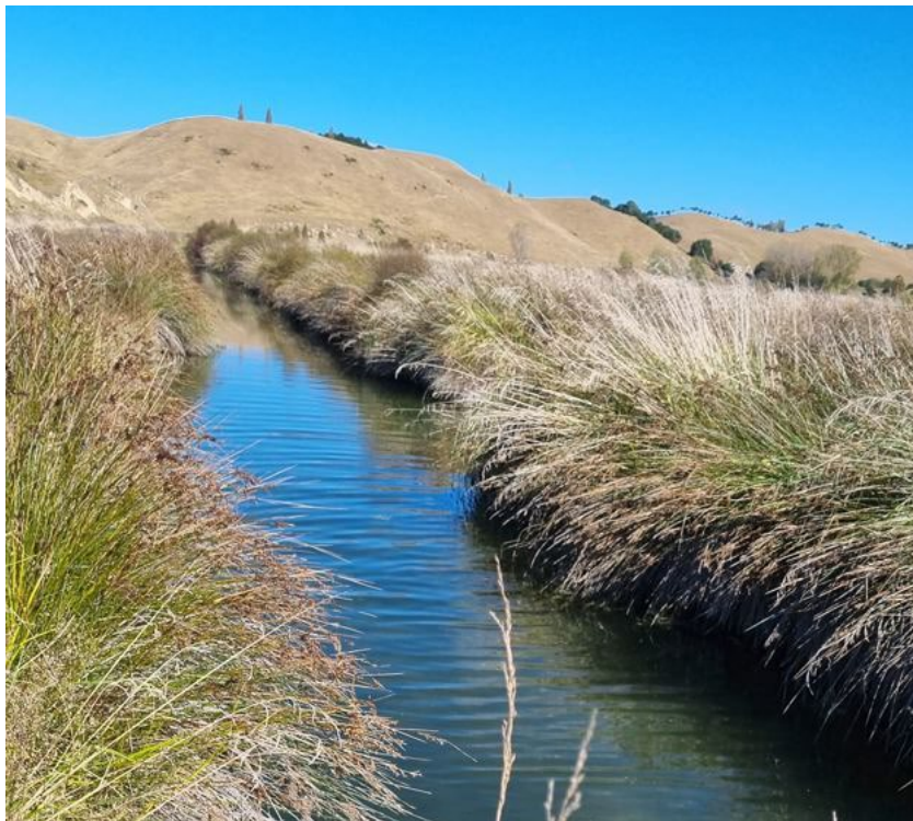
Photograph 15: T4 in dry weather facing upstream
