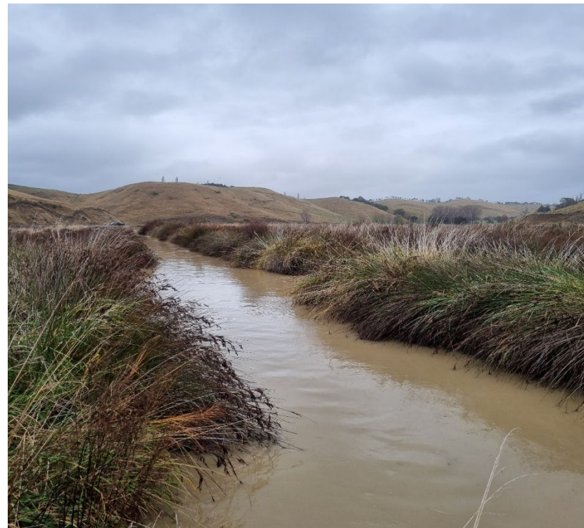
Photograph 16: T4 in wet weather facing upstream
